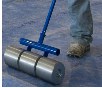
Embed sheet with roller
